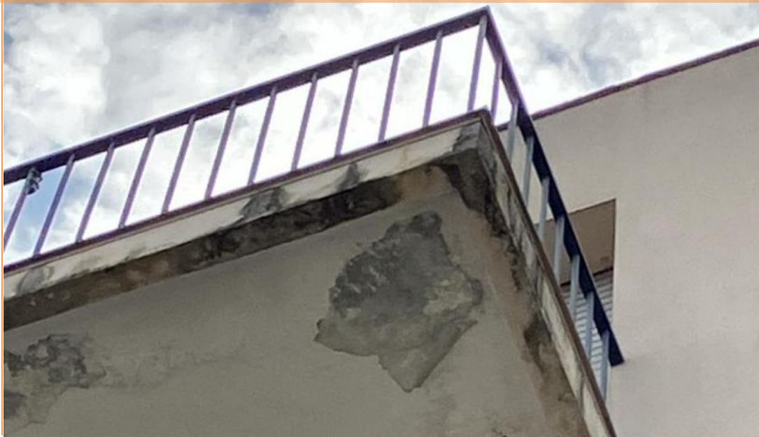
Poorly sealed balconies
